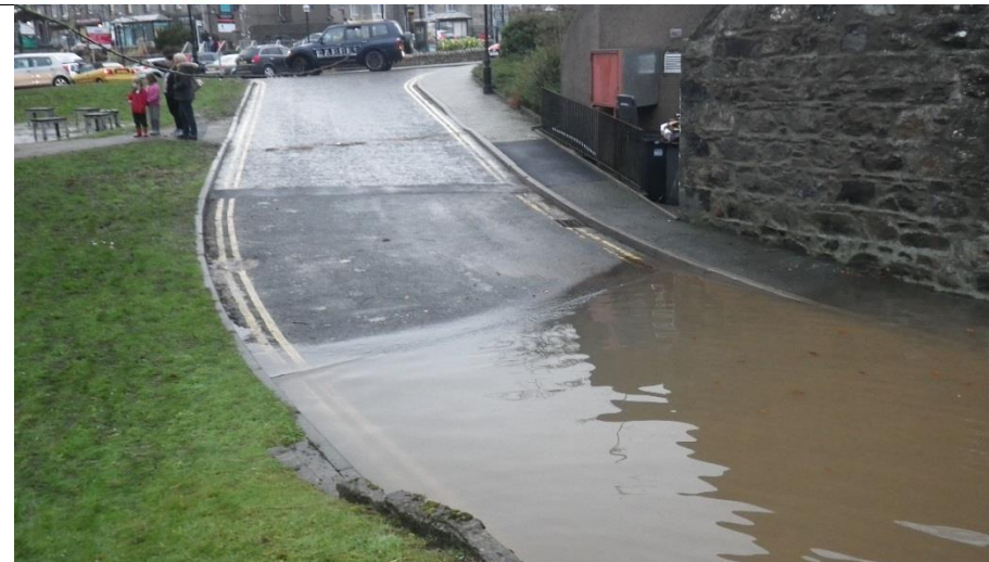
Photo 05: Road to Ythan Court looking West (taken 08/01/16)
