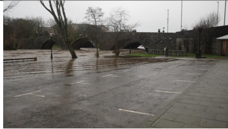
Photo 01: Market Street Car Park (taken 08/01/16)
