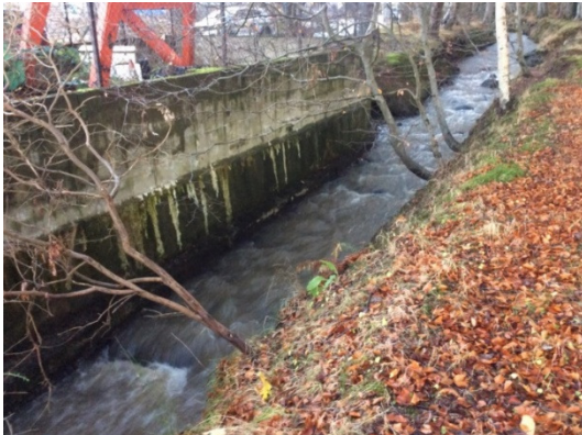
View from downstream of the wall showing water stains
