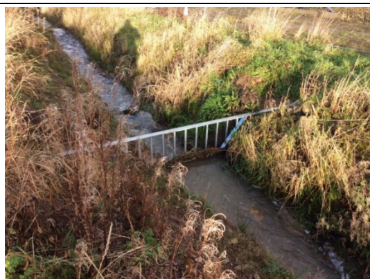
Trash screen upstream of culvert
