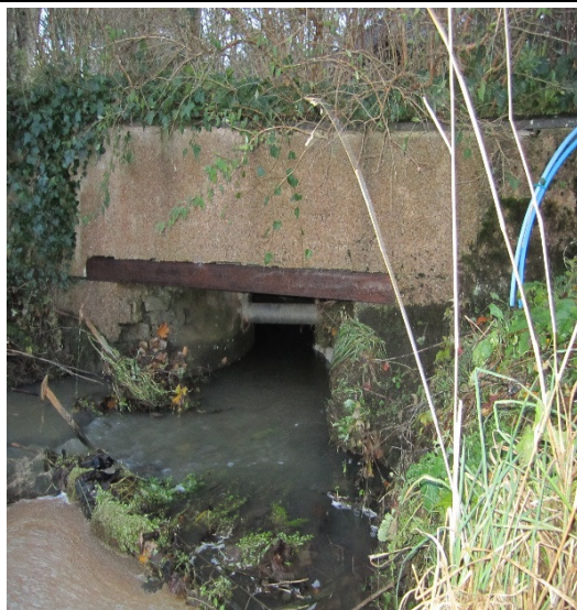
View from upstream of culvert. Service pipe inside culvert
